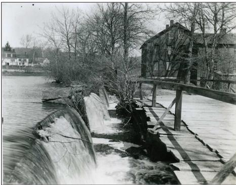
The triple-spillway dam at Falls River Cove in Essex once powered a gristmill, saw mill and iron forge at the Williams Family Complex & Shipyard, 1689-1845.
